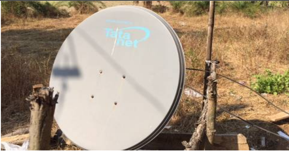
Figure 19: Vakrangee bears the Rs75000 investment on VSAT terminal
